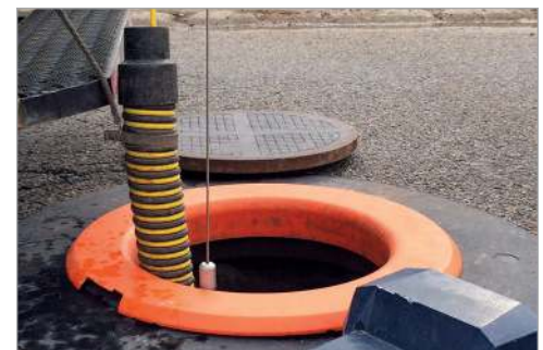
Sewer jet hose and camera protection
