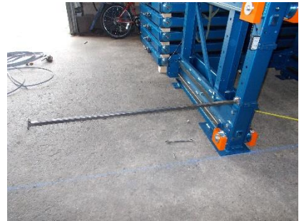
Bay temporary bracing
